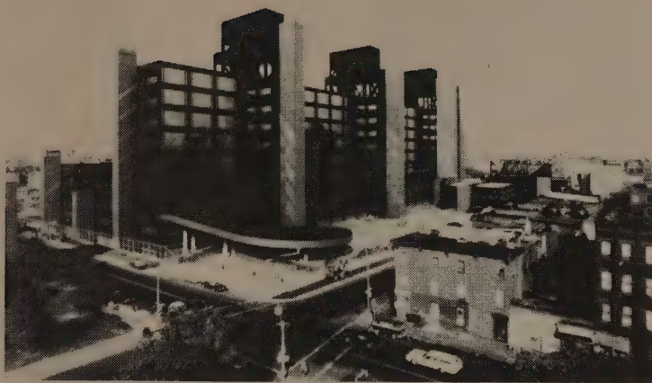
Woodhull Hospital, Brooklyn, NY. Kollman, McKinnel & Rosso & Sonder, architects.
